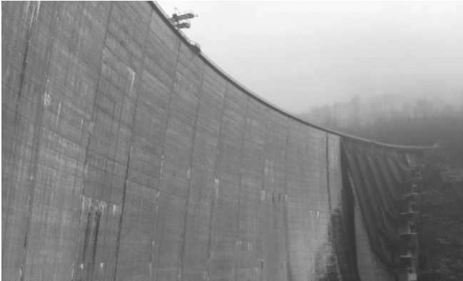
Verzasca dam (Switzerland): 220 m high arch dam
