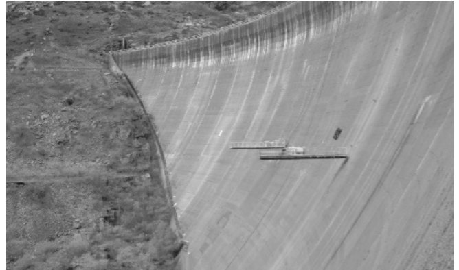
Pian Telesio dam (Italy): 80 m high arch-gravity dam affected by AAR
