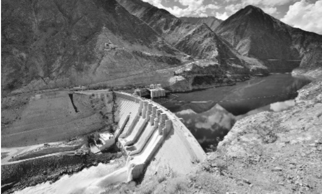
Cerro del Aguila (Peru): 88 m high gravity RCC dam
